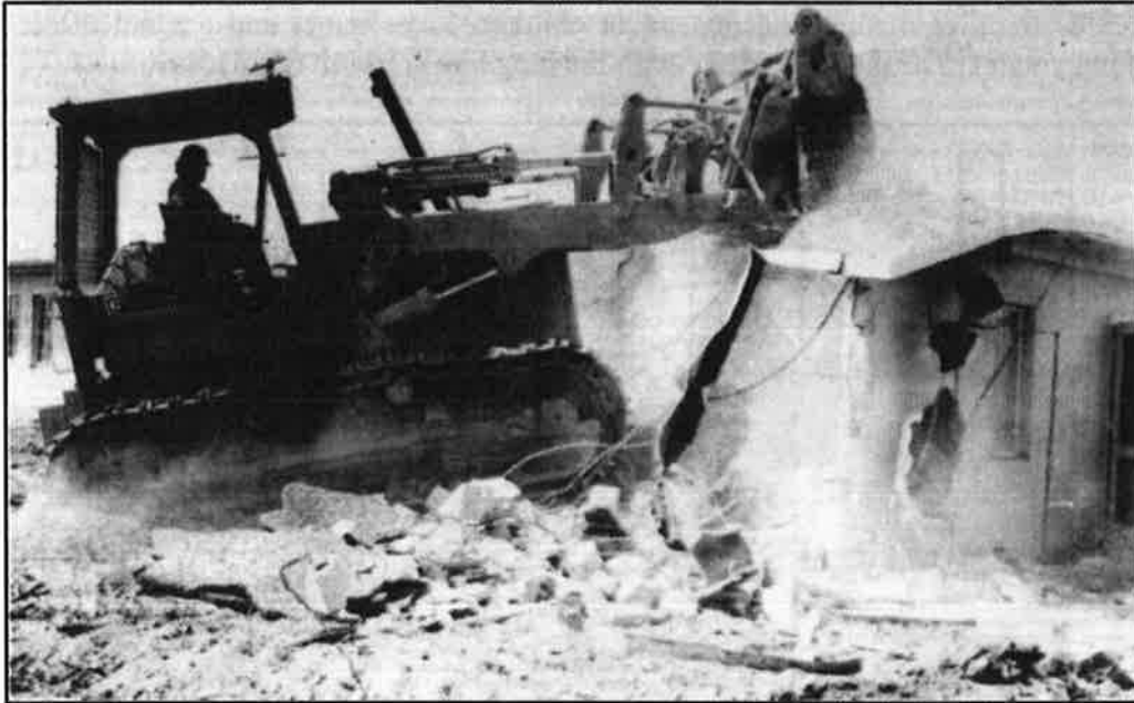
FIGURE 3. 1982 Demolition of 500 Navy Housing Units.
