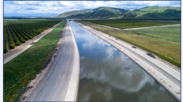
California Aqueduct (Kern County) Source: DWR, 2019
