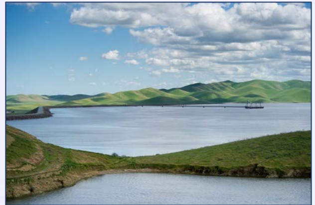
San Luis Reservoir (Merced County) Source: DWR, 2017
